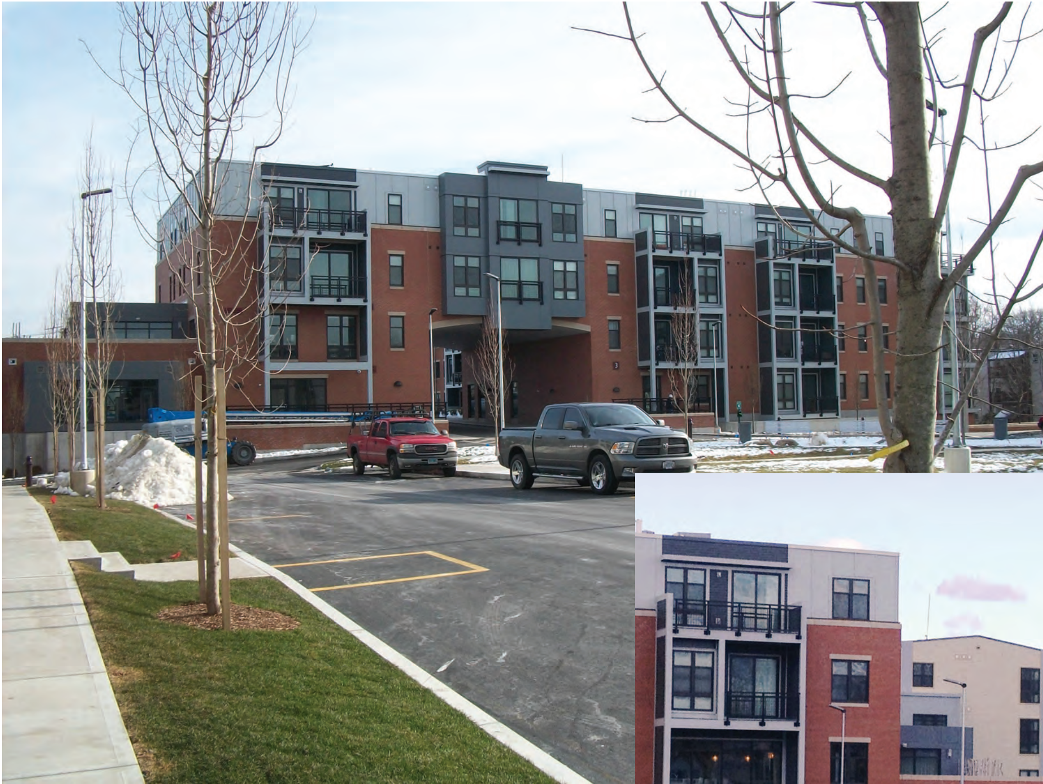
VIEW LOOKING EAST-From Building E
