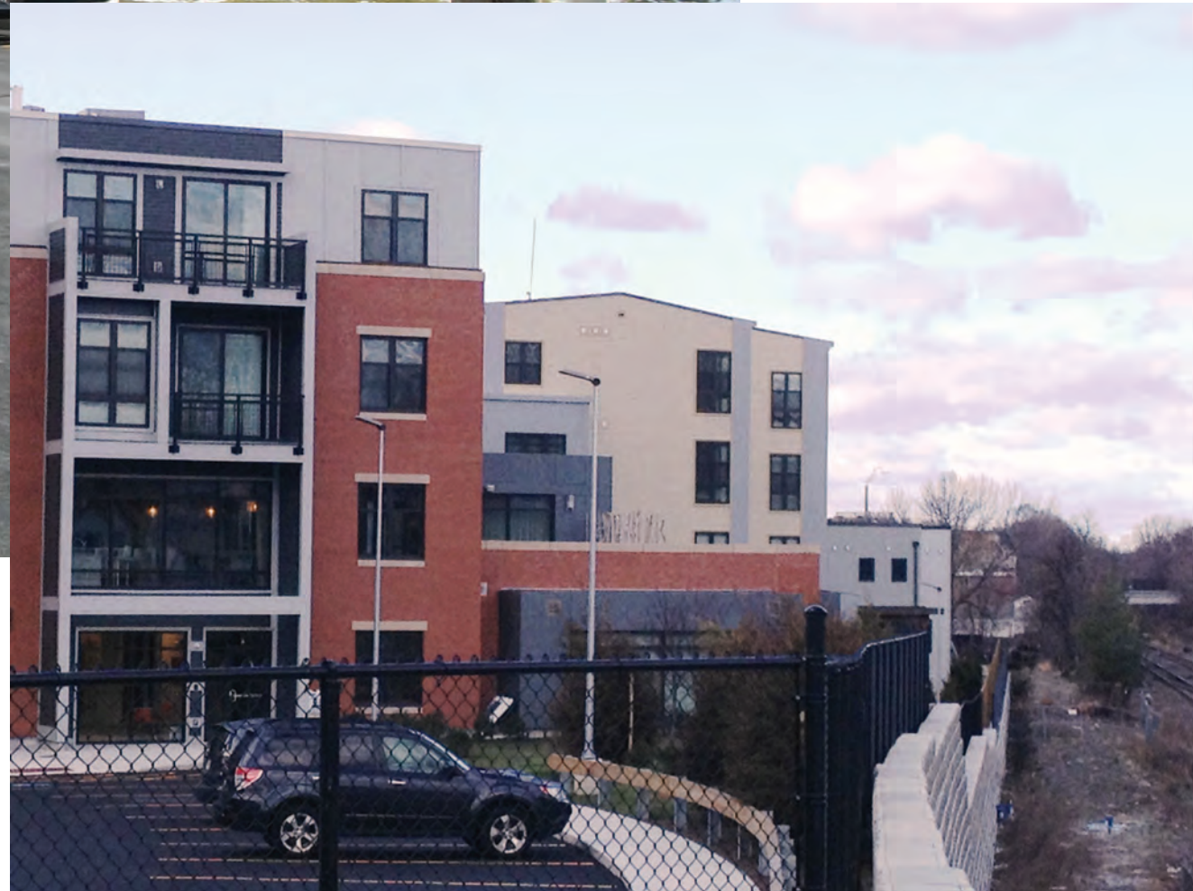
VIEW LOOKING WEST-From Lowell Street
