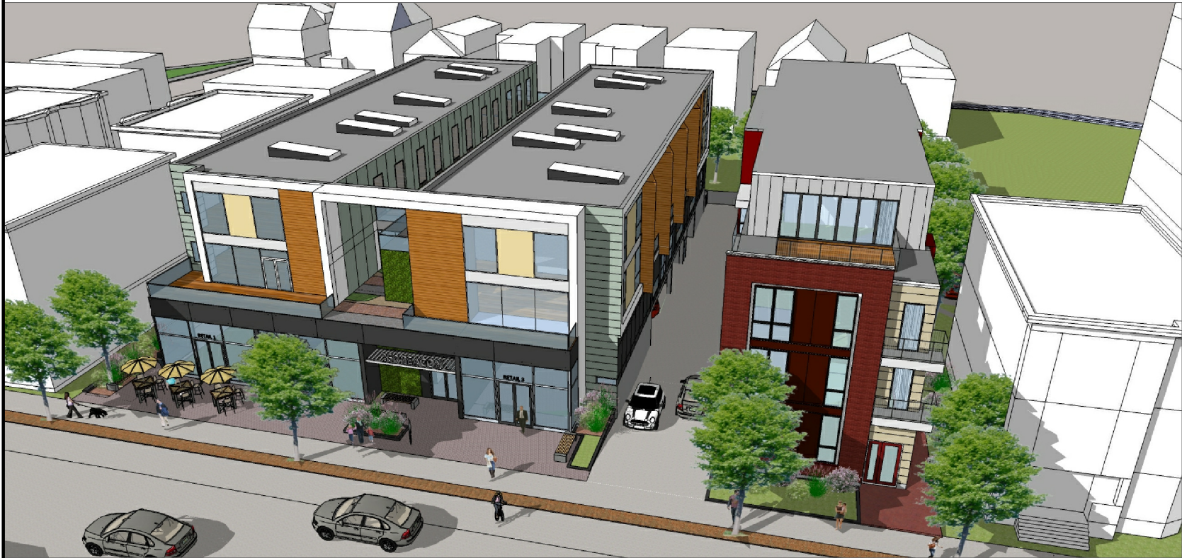
CONTEXT VIEW 260 AND 266 BEACON STREET
