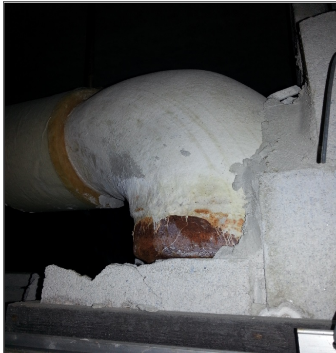
NON-Asbestos-Containing Roof Drain Insulation Above Suspended Ceilings Throughout School
