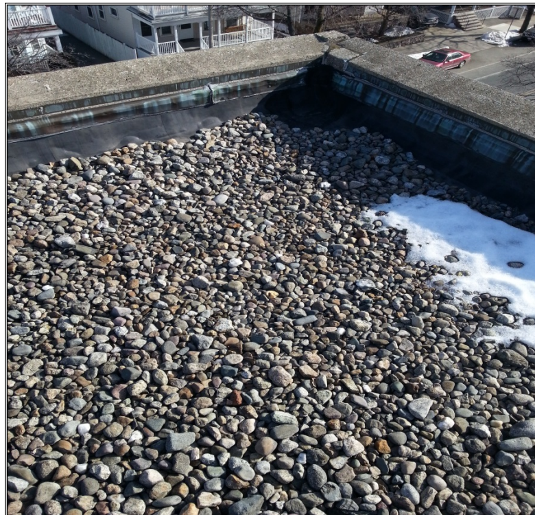
Typical Stone Ballasted Rubber Roof Over Multi-Layer Asbestos-Containing Roofing
