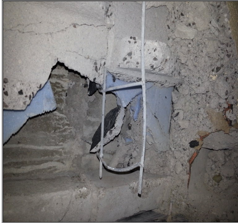
Asbestos-Containing Damp Proofing on Blue Foam in Insulation Board on Interior CMU Walls
