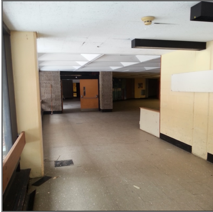
12"x12" Brown Asbestos-Containing Floor Tile and Mastic Located Throughout School
