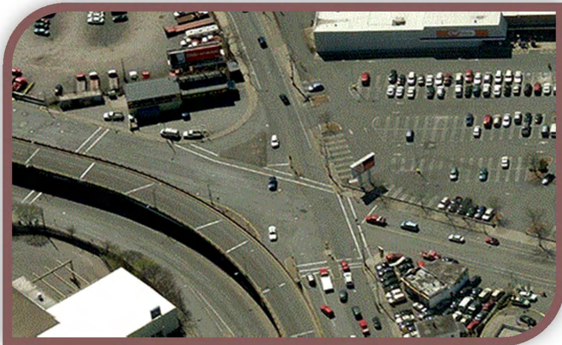
Intersection of Somerville Avenue and Medford Street at McGrath Highway
