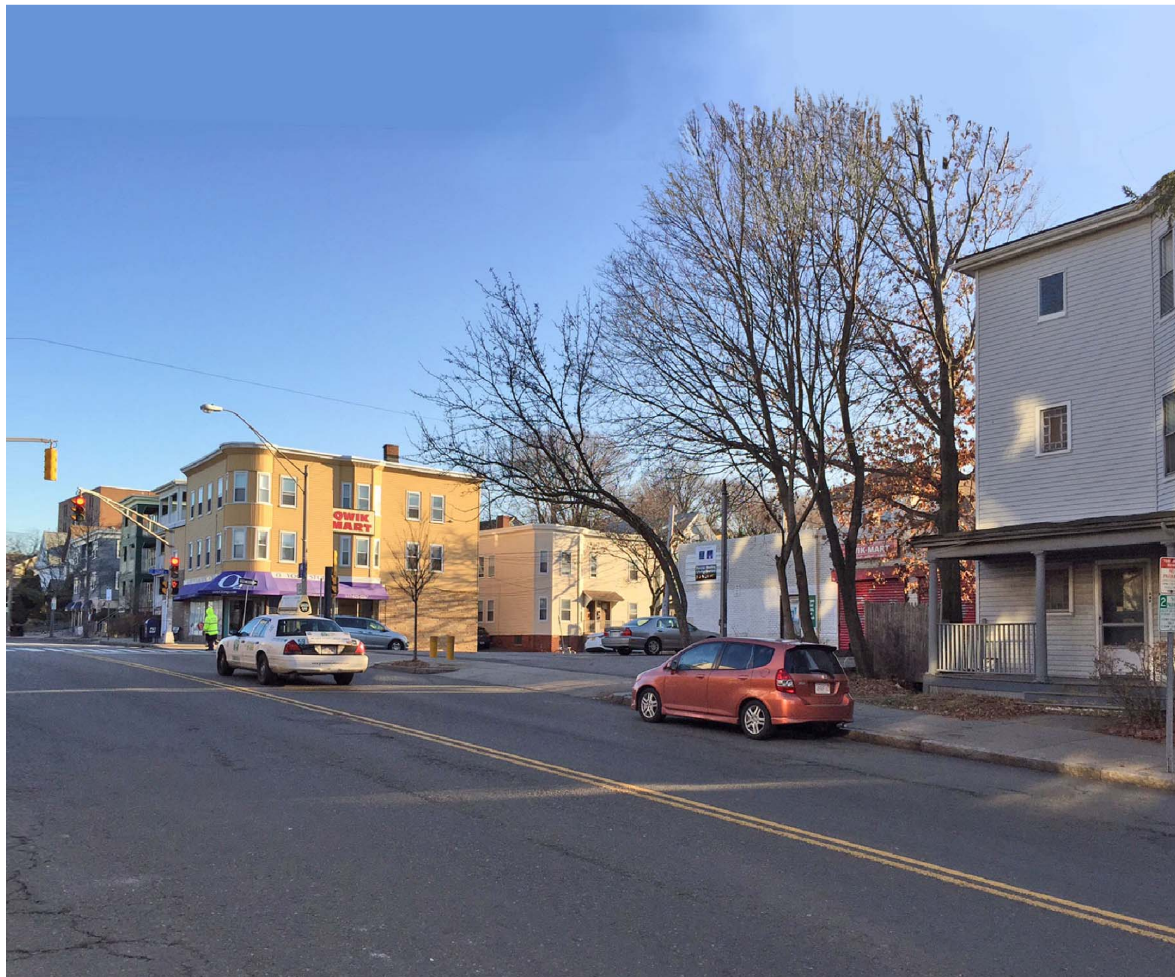
EXISTING VIEW FROM HIGHLAND AVE
