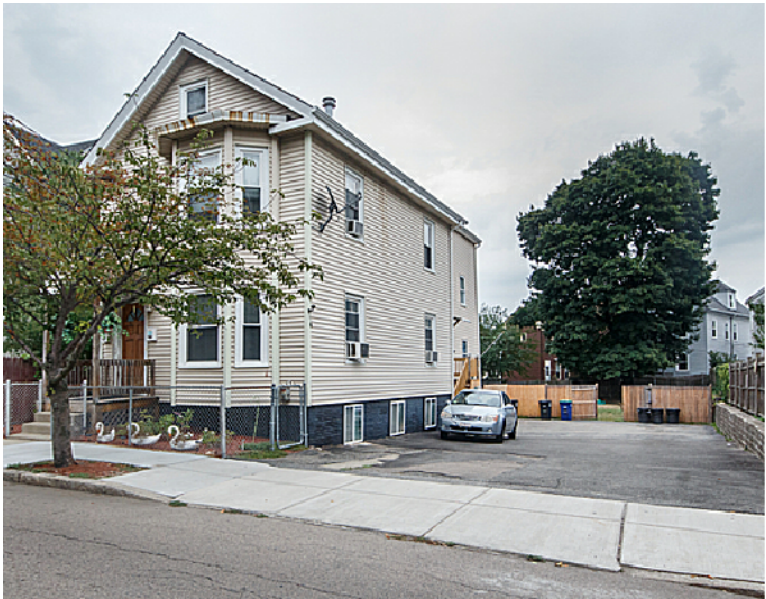
FRONT YARD VIEW
