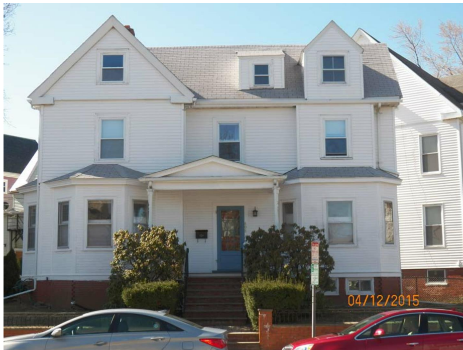
NORTH ELEVATION VIEW FROM BROADWAY
