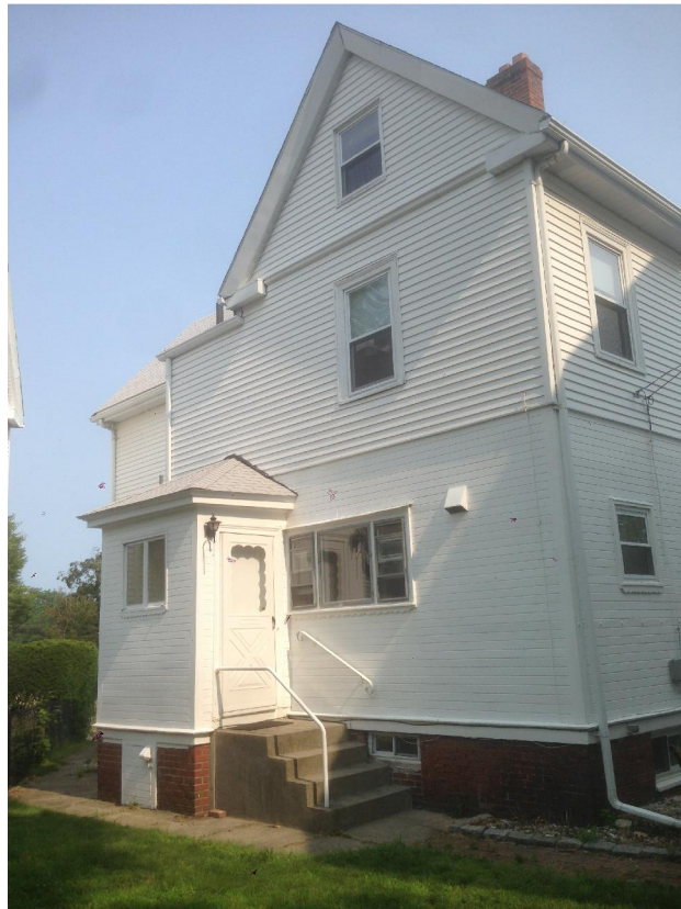
SOUTHEAST ELEVATION REAR
