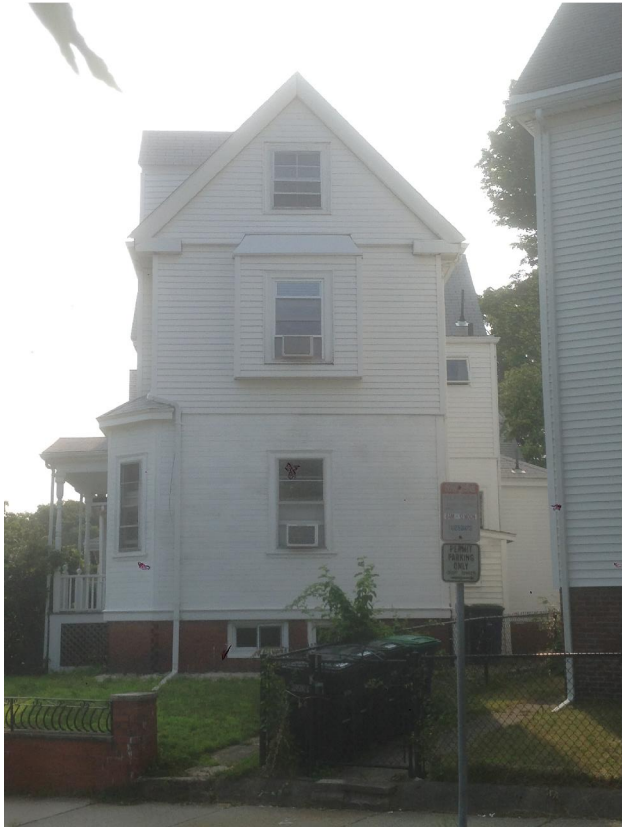
WEST ELEVATION VIEW FROM BILLINGHAM ST
