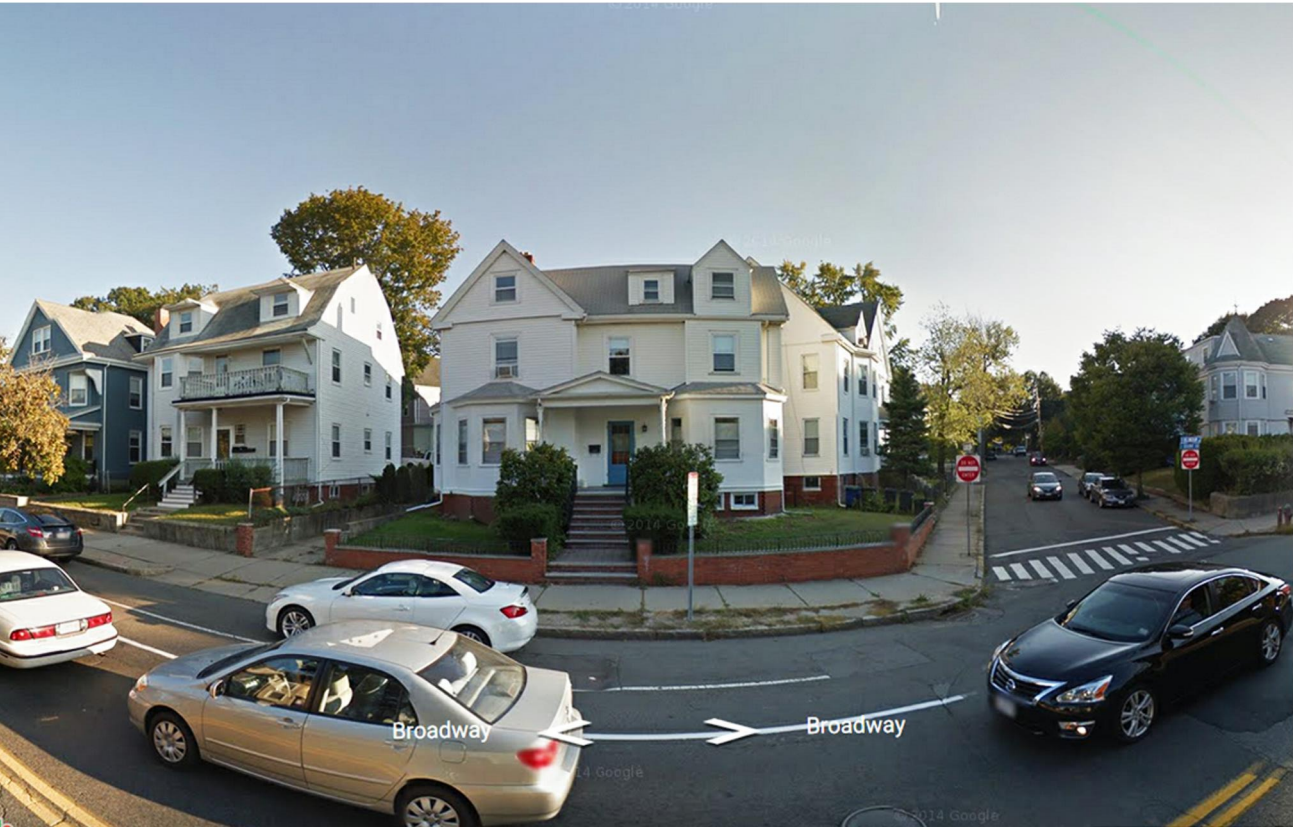
NORTH ELEVATION VIEW FROM BROADWAY
