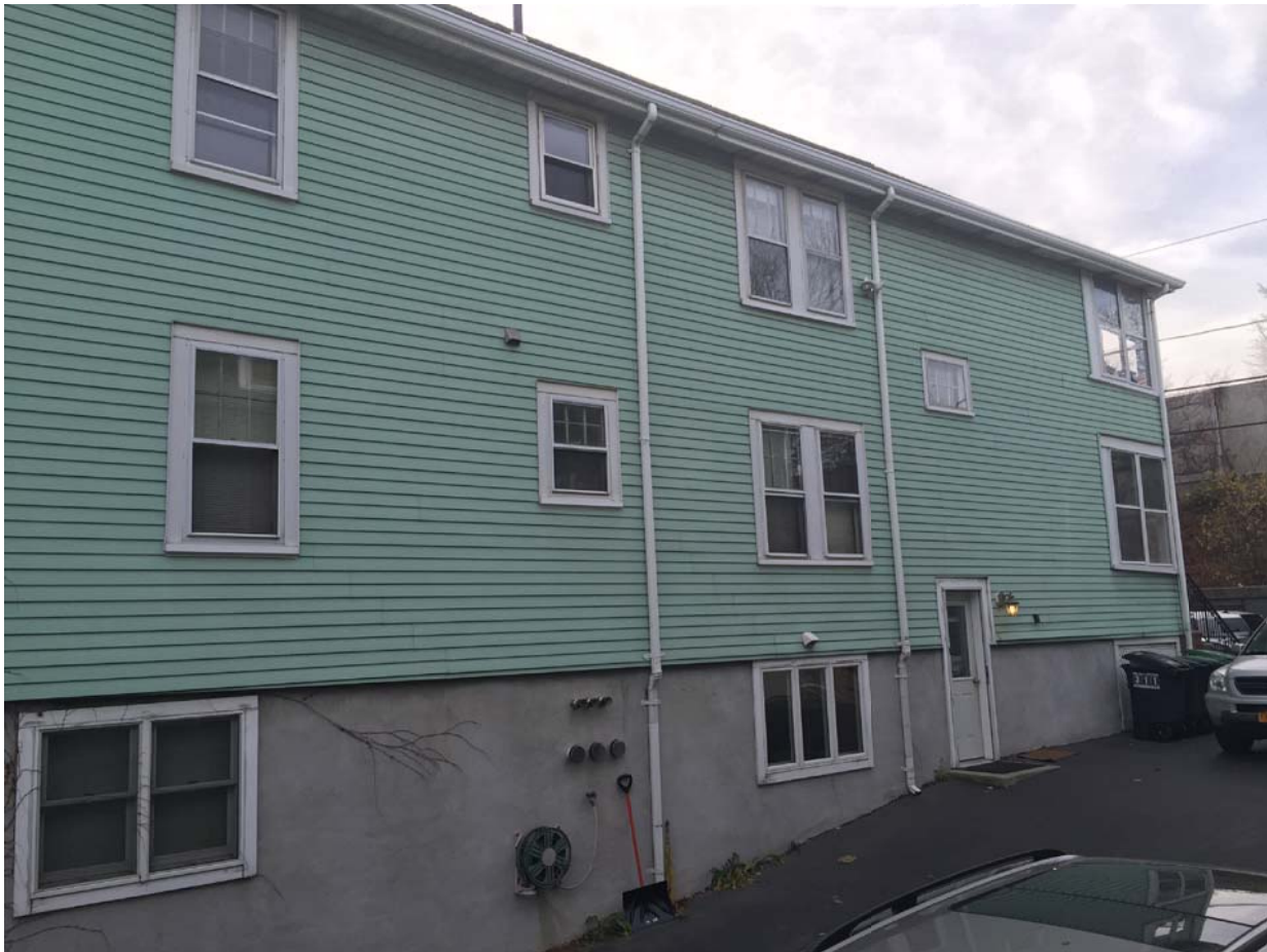
SIDE VIEW FROM NORTHEAST
