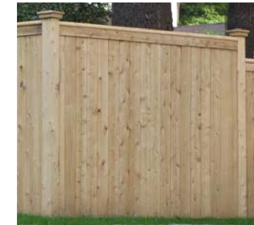
solid board fence | 6' ht. along west property line in rear yard | 3' ht. along west property line between residences | 4' ht. along carpark on east property line
