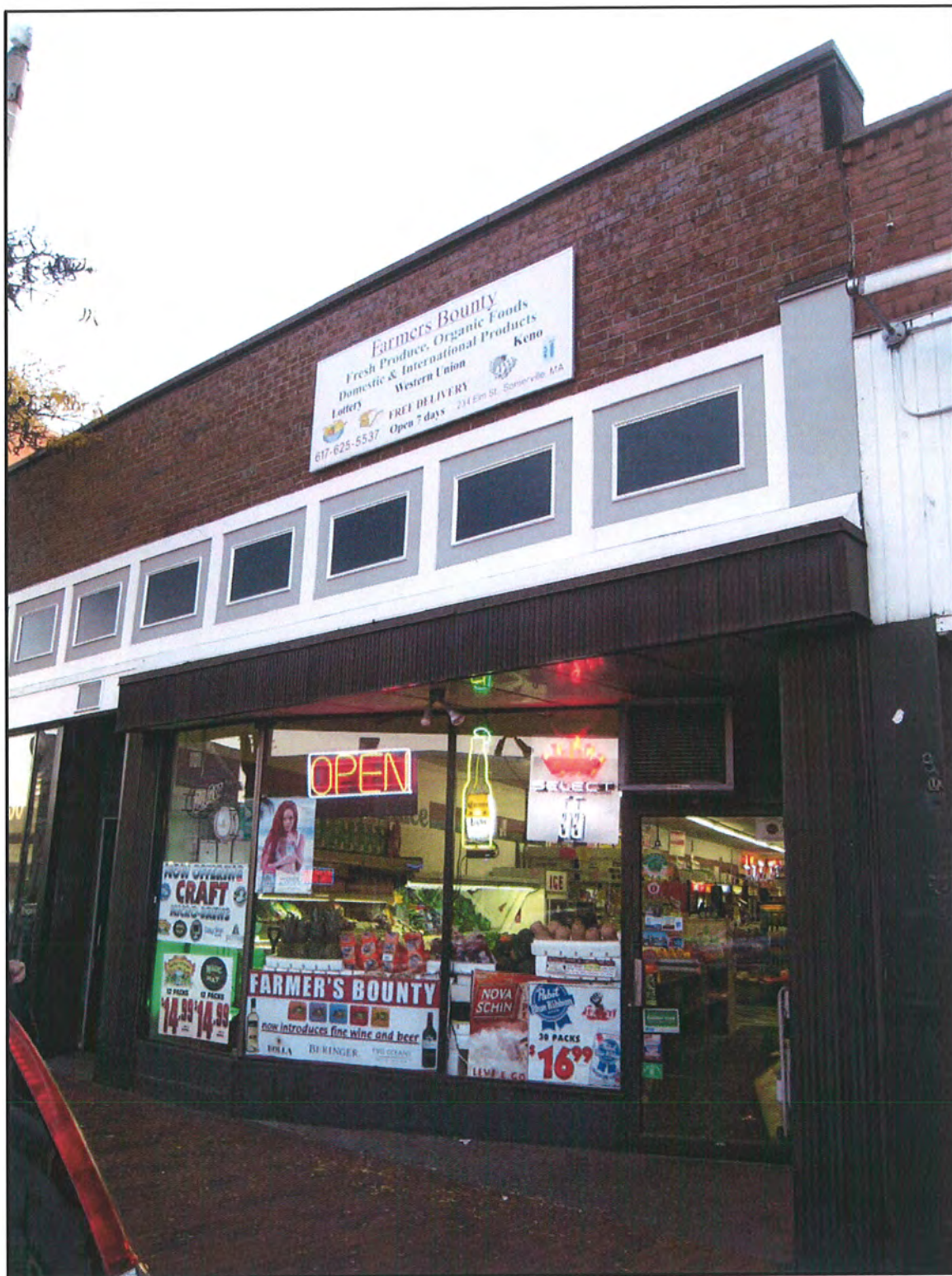
Existing Storefront View from Elm Street
