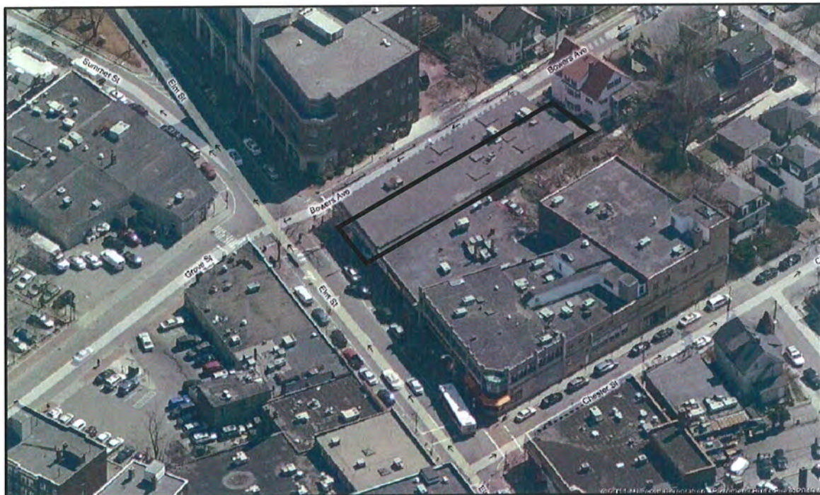
Aerial View — Facing Southeast
