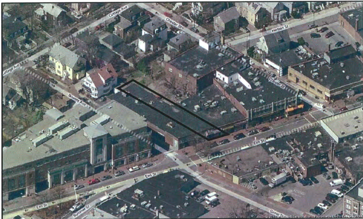
Aerial View — Facing Southwest
