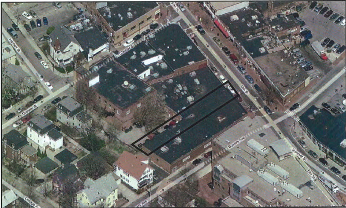
Aerial View — Facing Northwest
