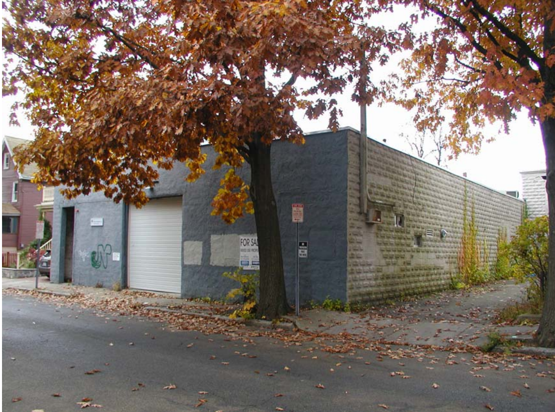
Existing Conditions on Elmwood Street
