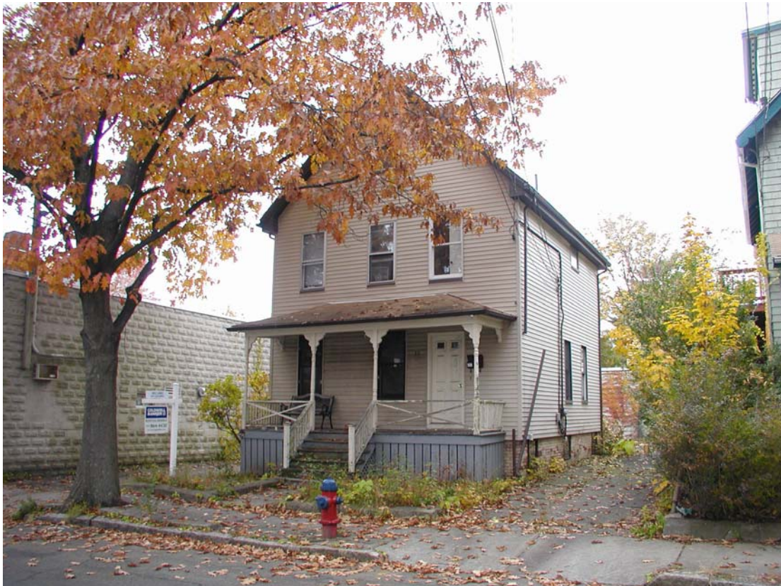
Existing Conditions on Elmwood Street
