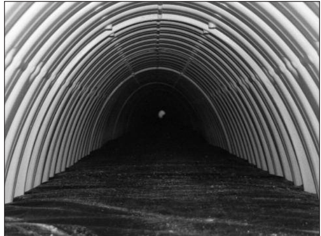
Looking down the Isolator Row.
