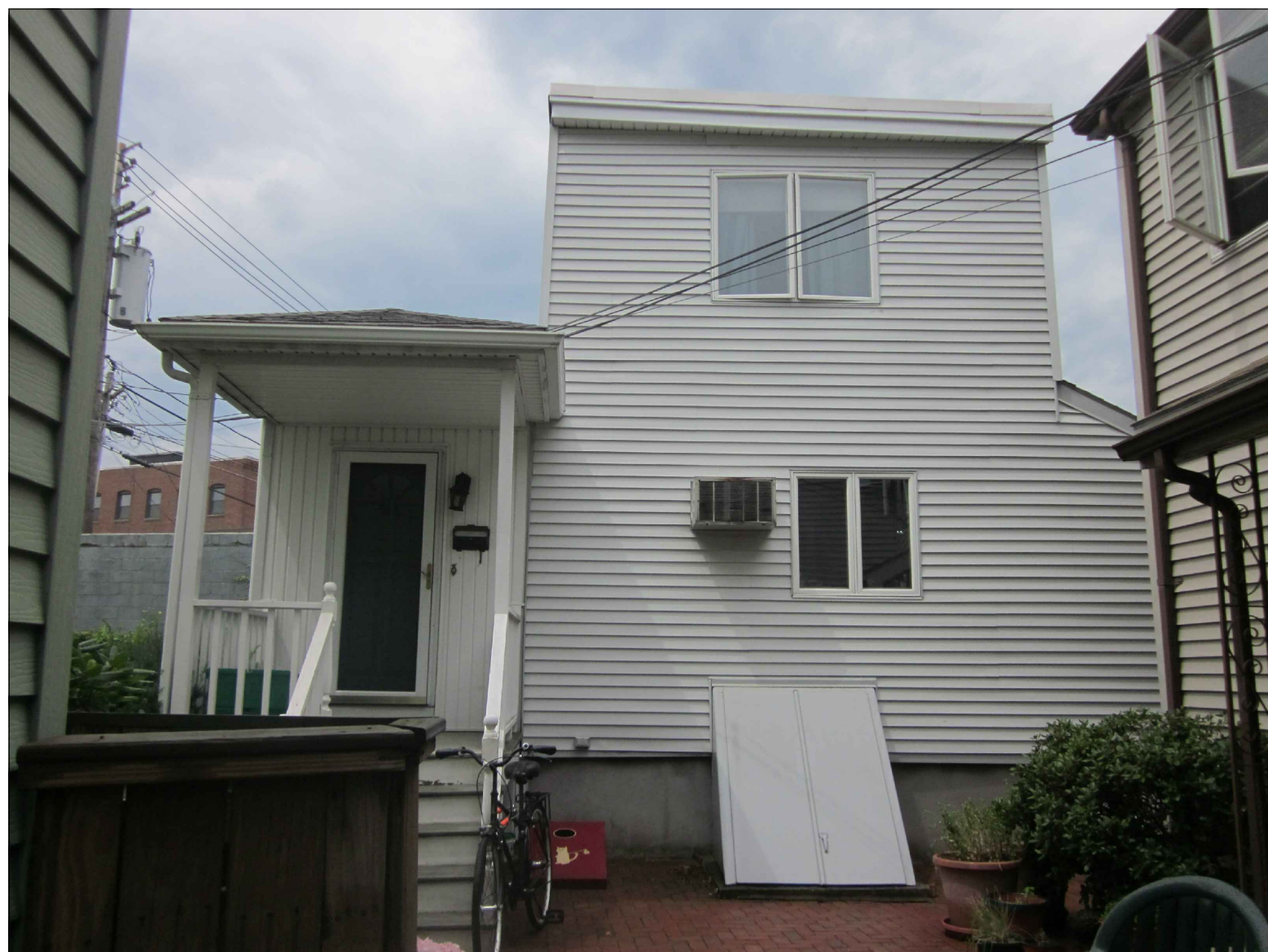
3a Front Elevation Photo Existing from courtyard
