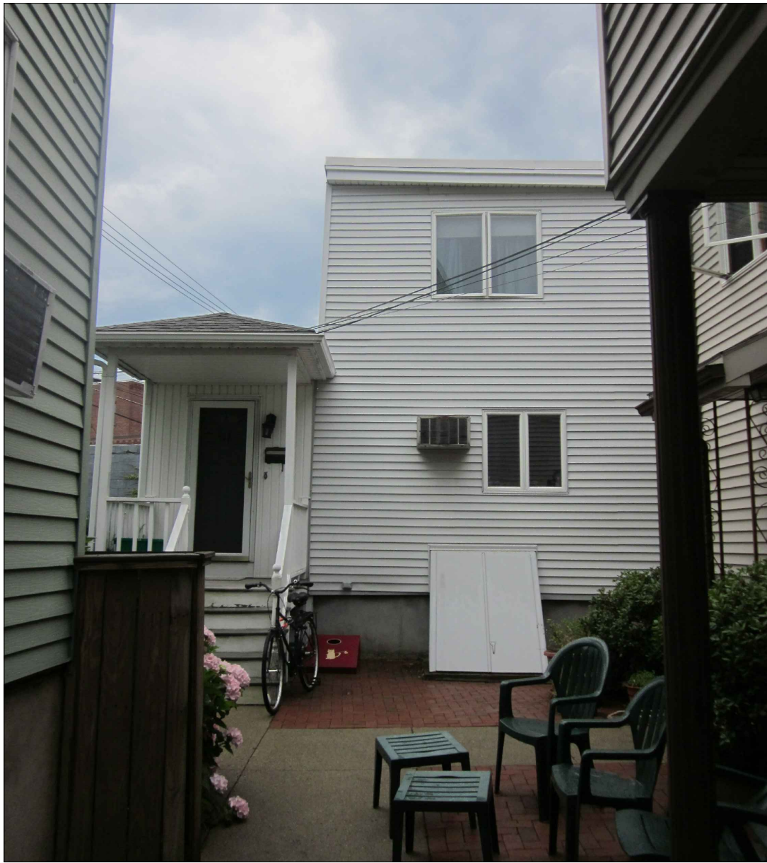
Front Elevation Photo Existing 52A Medford St.
