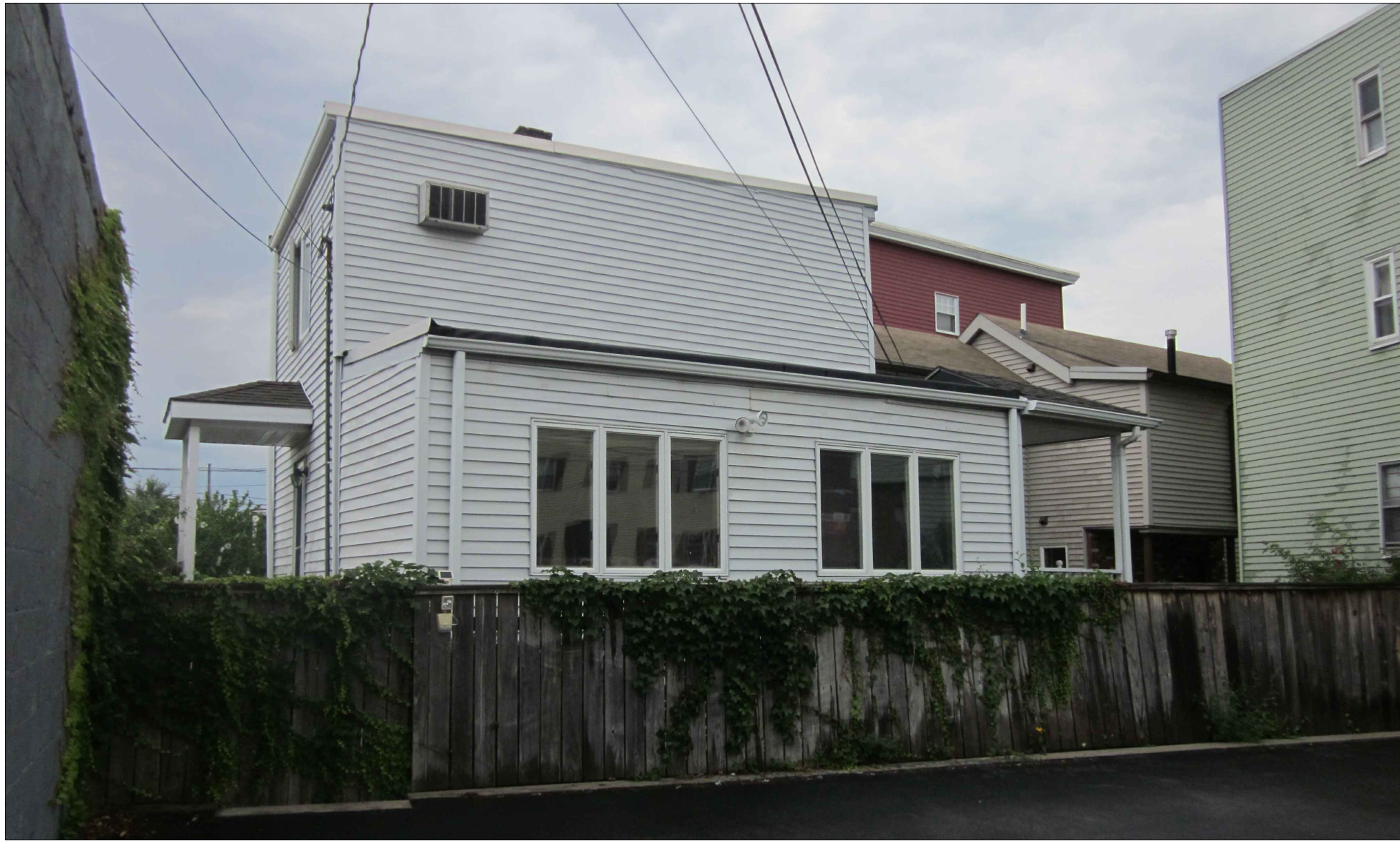
Side Elevation Photo Existing 52A Medford St.
