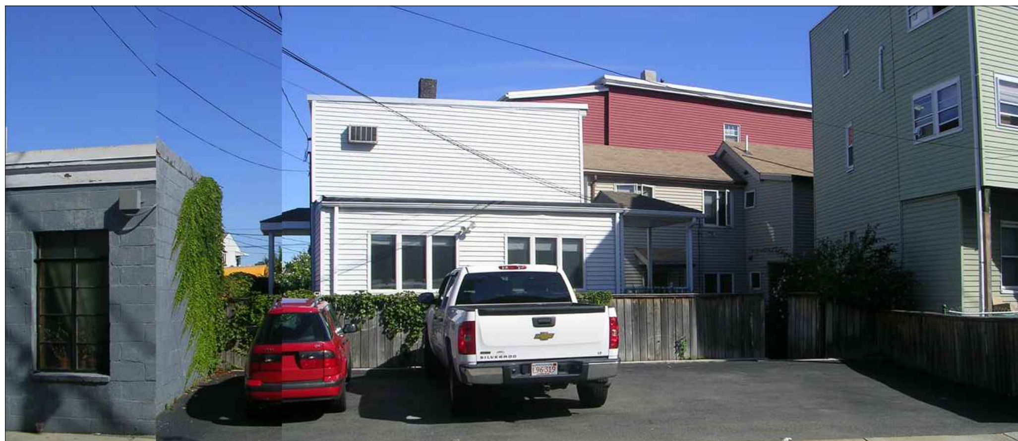
2 Side Elevation Photo Existing
