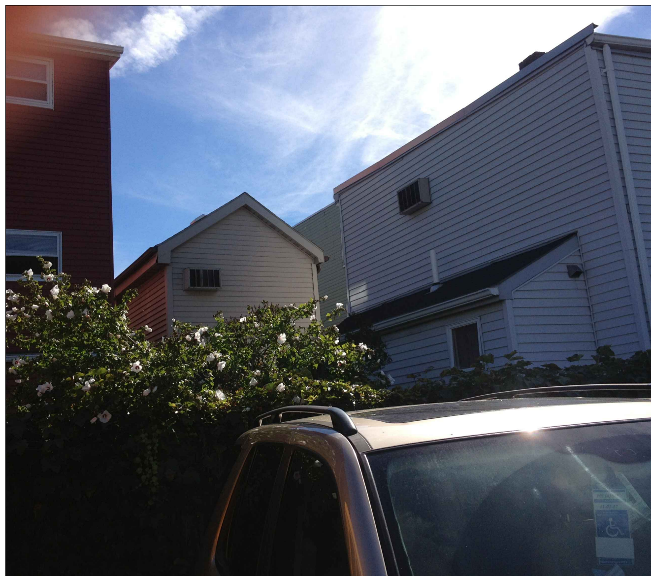
4 Side Elevation Photo Existing
