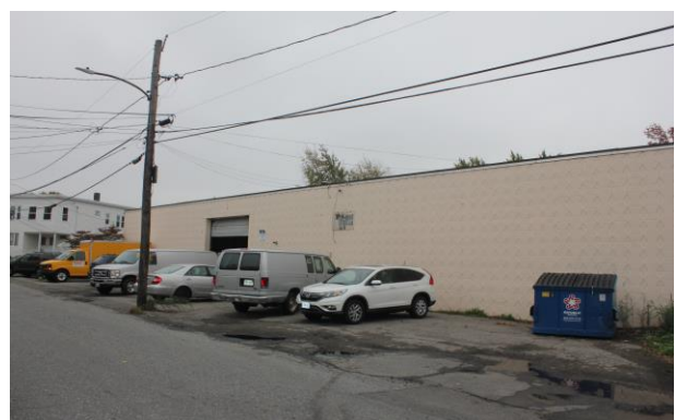
Street view of Murdock Street
