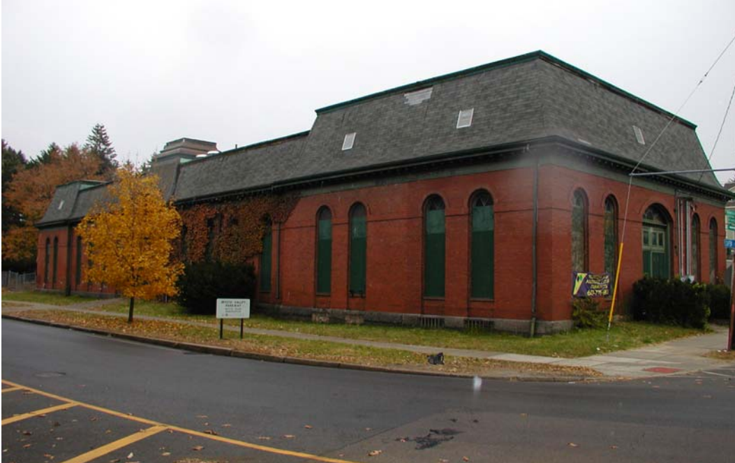
Existing Condition of Pump House Building
