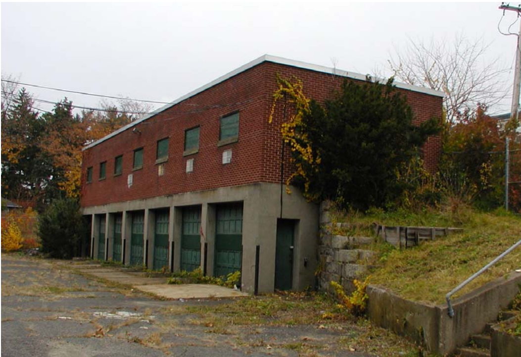
Existing Condition of Office/Garage Outbuilding
