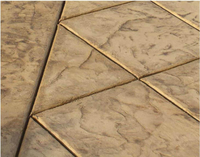
Concrete Paving | Integral Color & Stamped Pattern
