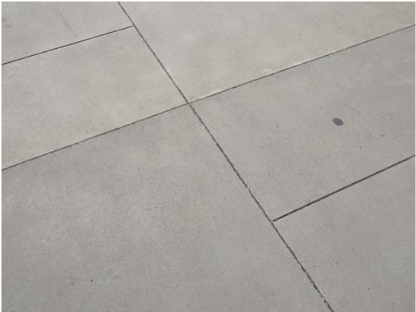
Concrete Paving | Sawcut Scoring Pattern
