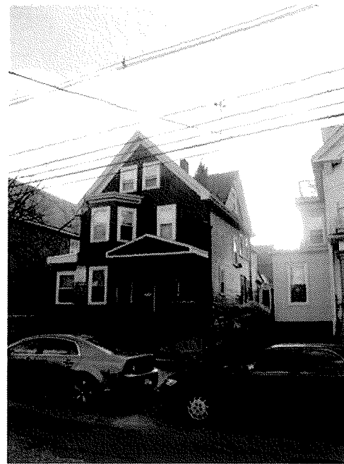
NORTHEAST CORNER OF MAIN HOUSE
