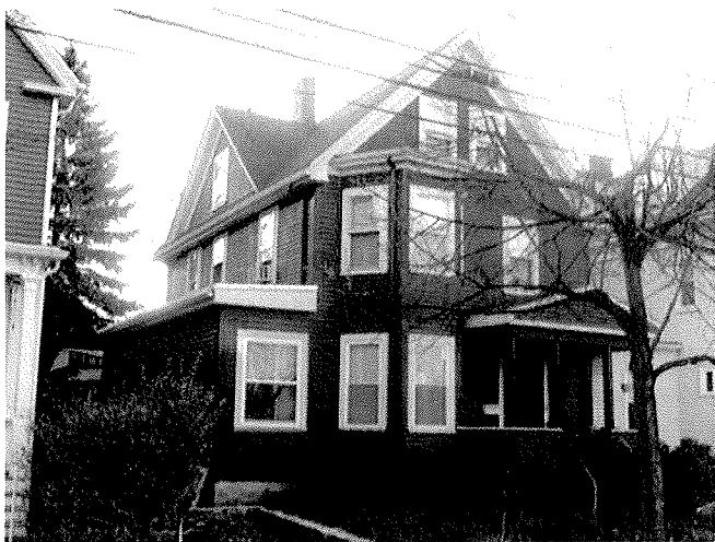
NORTHWEST CORNER OF MAIN HOUSE
