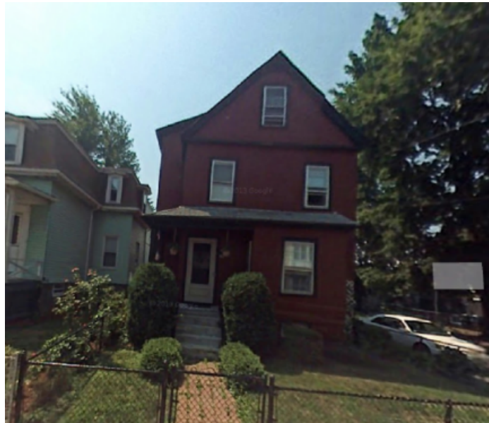
FRONT YARD VIEW
