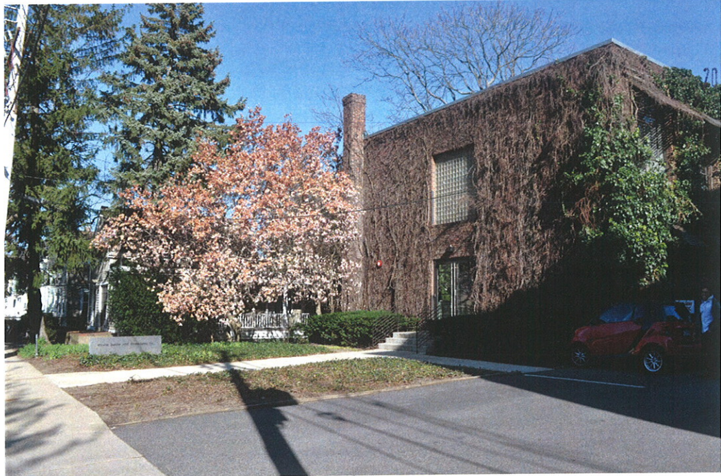
CURRENT VIEW FROM NORTH-EAST
