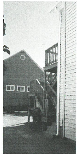
③ REAR EXTERIOR STAIRS - EXISTING NOT TO SCALE
