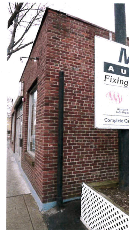
EX. CONDITIONS, POLE, MIKE'S AUTOMOTIVE DRIVEWAY
