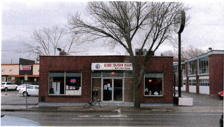
FACADE, EXISTING CONDITION
