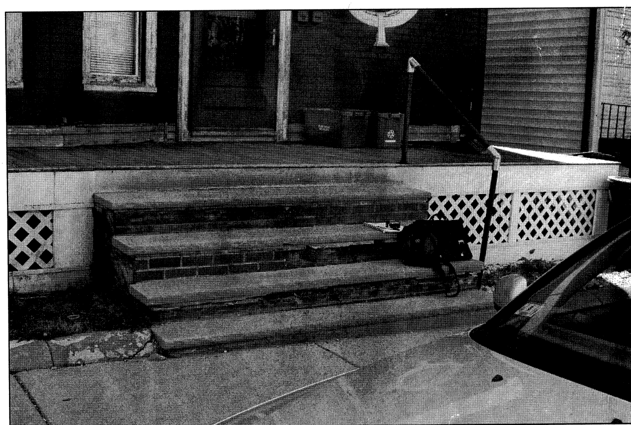
FRONT VIEW (SYCAMORE ST.)
