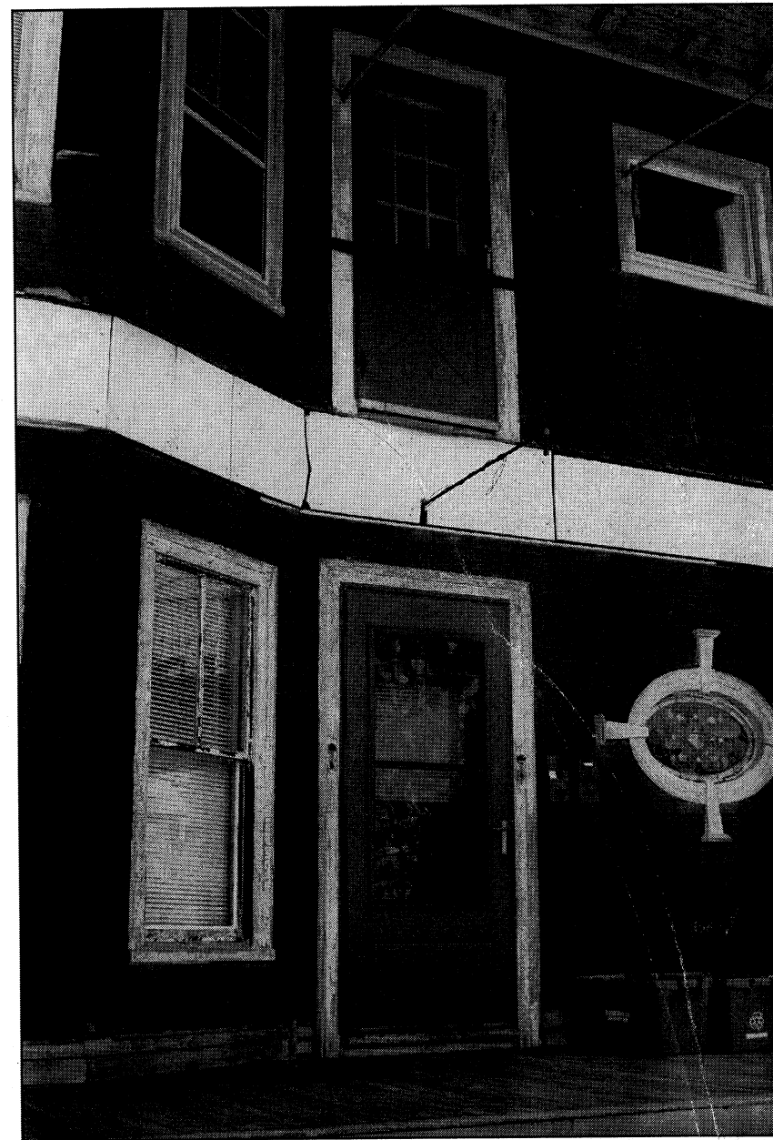
FRONT VIEW (SYCAMORE ST.)
