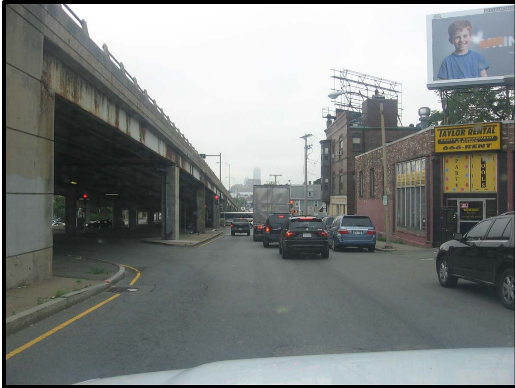
McGrath Highway Southbound Approach Note Excessive queuing
