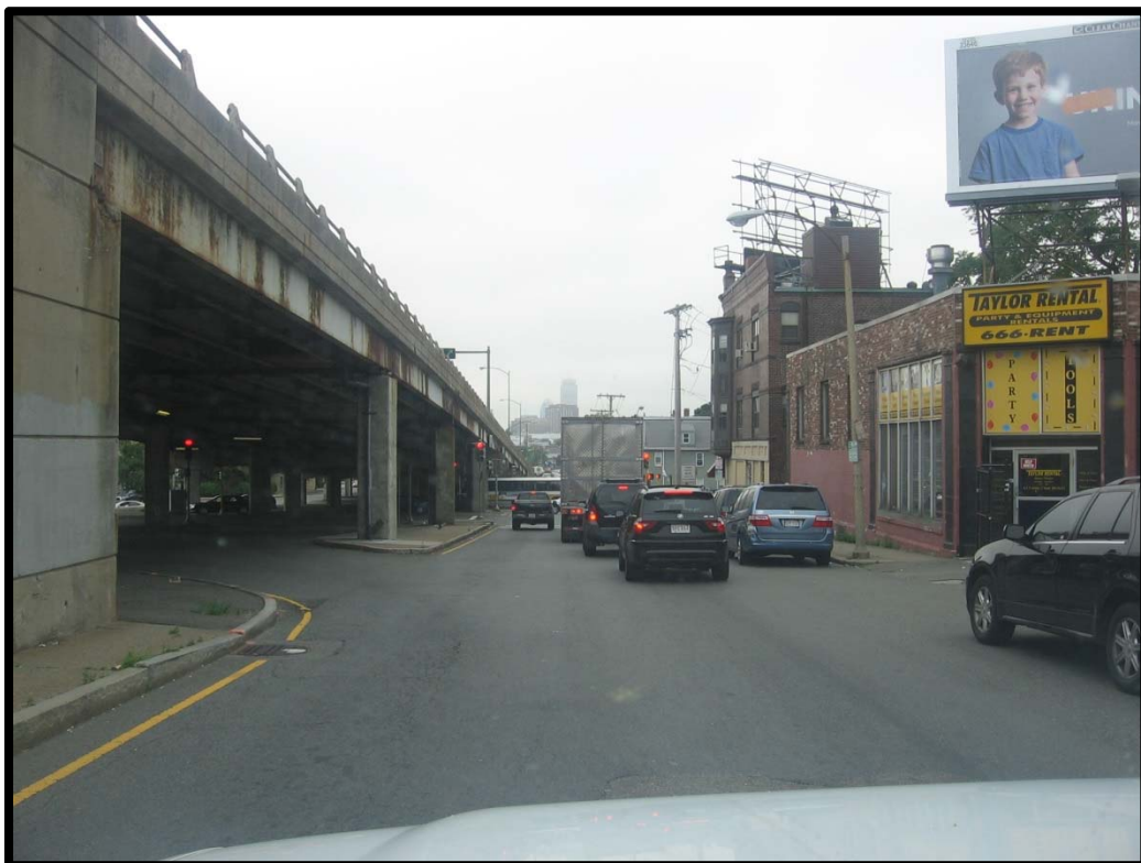
McGrath Highway Southbound Approach Note Excessive queuing
