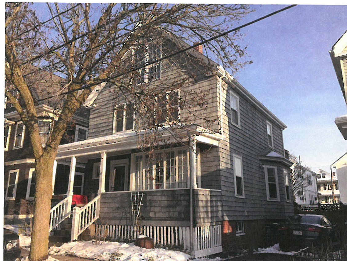
STREET VIEW FROM WEST
