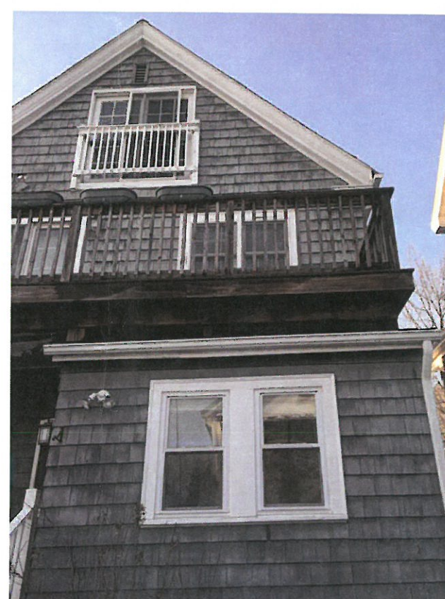
PARTIAL REAR VIEW FROM EAST
