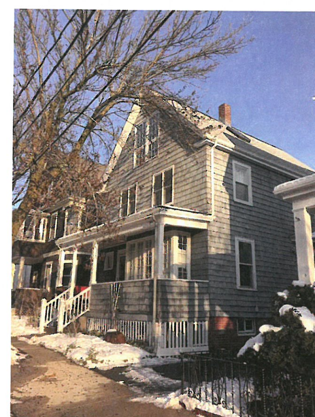
STREET VIEW FROM SOUTHWEST
