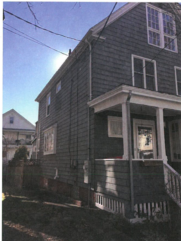
SIDE VIEW FROM NORTHWEST
