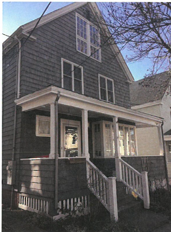
44 VICTORIA STREET - STREET VIEW
