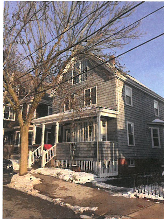
44 VICTORIA STREET - STREET VIEW
