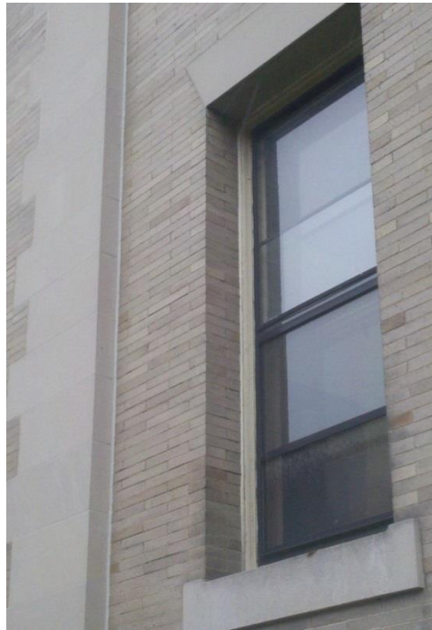
Window and joint caulking
