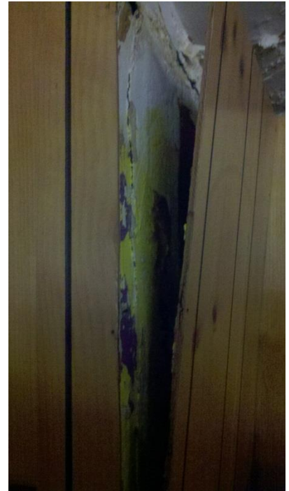
Suspect lead-based paint
