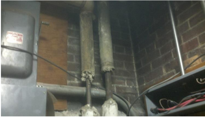
Asbestos insulation
