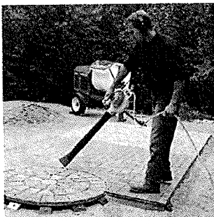
Figure 6. Whether using liquid or dry joint stabilization materials, the surface of the pavers should be cleaned with a blower or broom after the joint sand is compacted into the joints.
