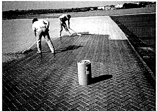
Figure 10. Urethane is applied with squeegees to stabilize joint sand between pavers on aircraft pavement.
