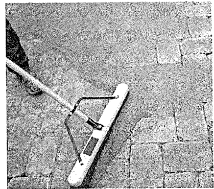
Figure 5. Joint sand can be pre-mixed and delivered to the site (typically in bags), or mixed with stabilizer at the site, then swept into the joints, compacted for consolidation in them to create interlock, and wetted to activate the stabilizer.
