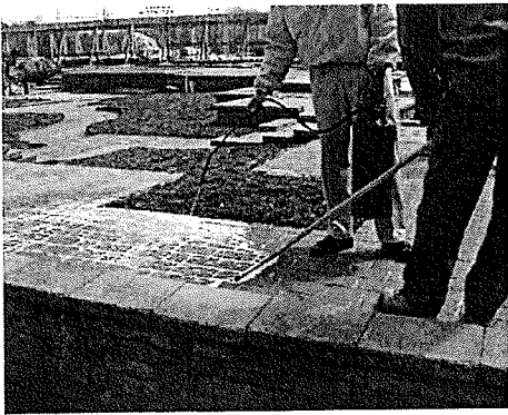
Figure 3. This liquid joint sand stabilizer is applied with a low-pressure sprayer and squeegeed across the surface after allowing some time for soaking into the joints. This helps maintain slip and skid resistance of the paver surface.
