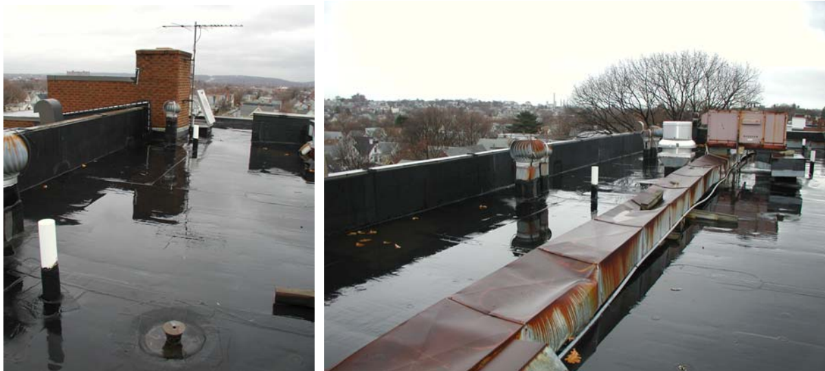
Existing chimney /location of stealth chimney (bottom left), Roof top and parapet (bottom right)
