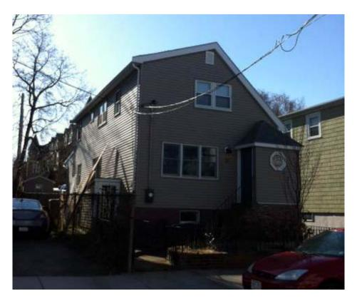
2. <u>Proposal:</u> The proposal is to bring the two entryways to code and make them more practical. The front entry will have a new roof that is an asymmetrical gable that extends over a landing. The stairs will be reoriented so that they lead from this landing straight to the sidewalk. The reconfiguration of the front steps will allow for more than 50 sf of additional green space in the front yard.
