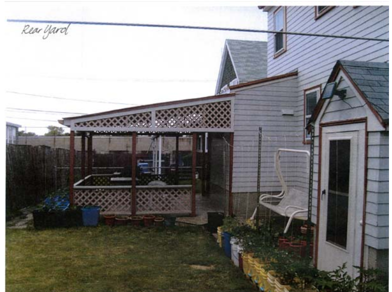
Left Photo – Egress along narrow side yard, porch, and porch roof. Existing stairs will be demolished. Above Photo – Rear Yard showing the existing basement entrance, the 1-story addition, and existing porch and roof. The existing roof will be demolished.
