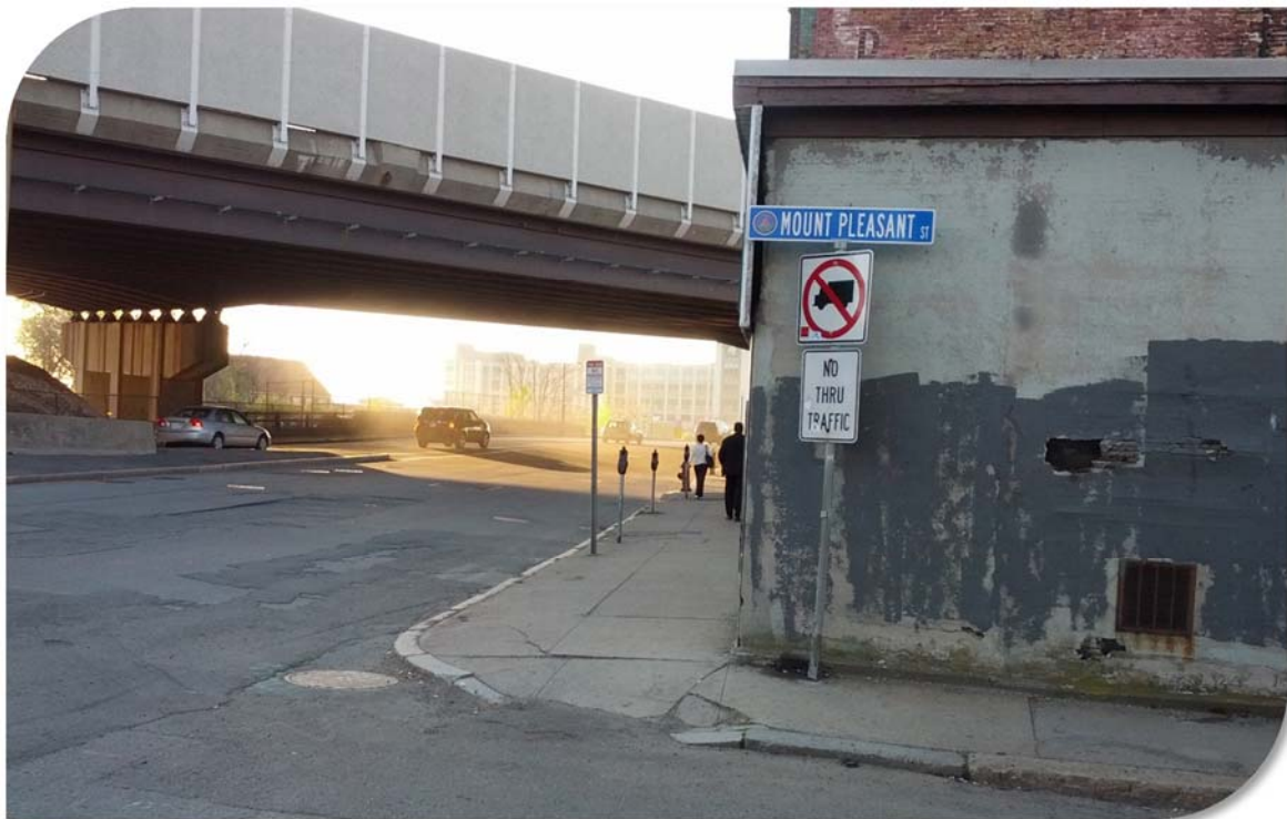
Broadway at Mount Pleasant Street, looking east at the project site
